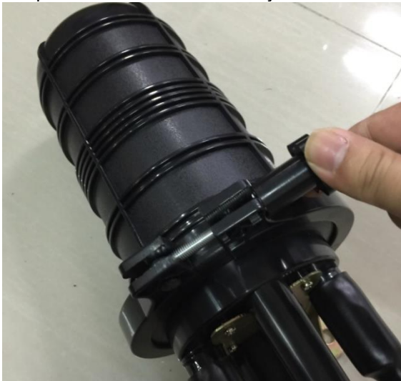
9. Attach the splice tray cover, rotate the hoop, and compress it.
