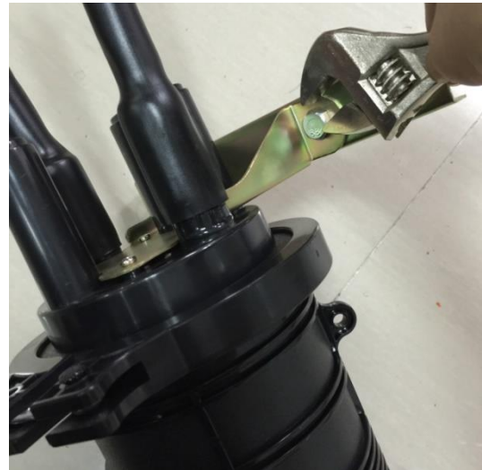
10. Attach the hanging hook with a wrench.
